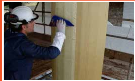
DEFECT REMEDIATION / BLAST MITIGATION
